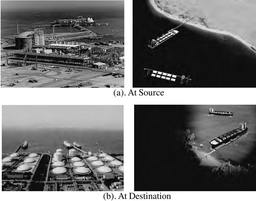
Figure 5-7 Loading and offloading terminal for LNG and CNG (XGAS website http://www.xgas.us )
